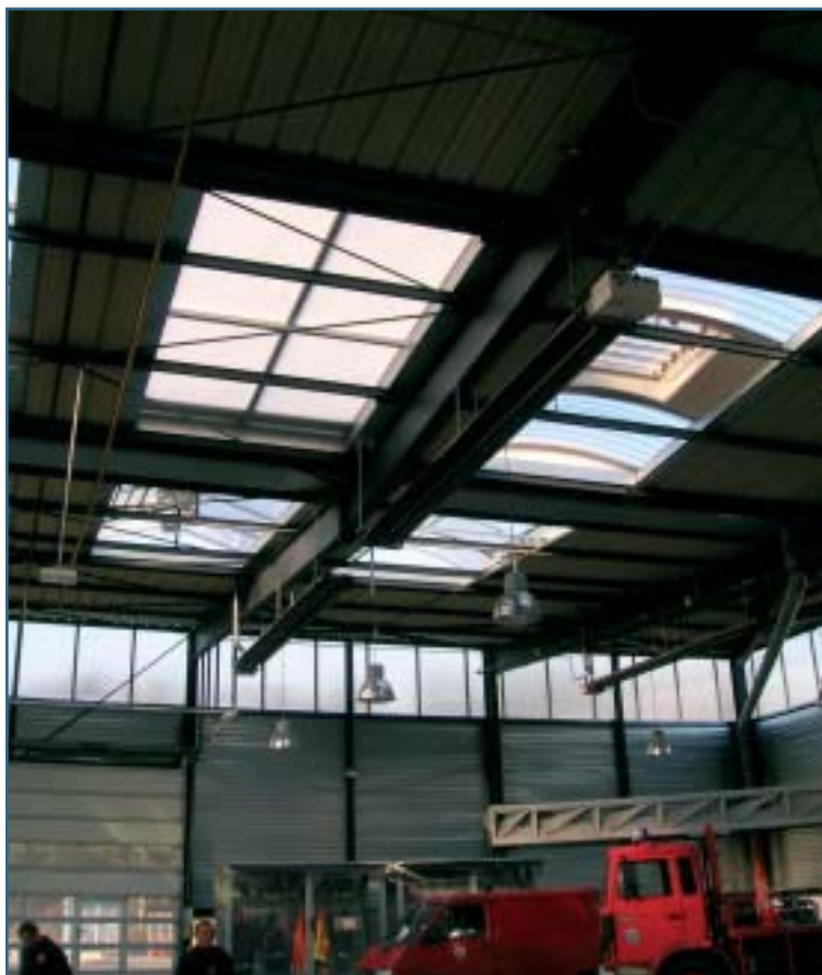
Thermoclear 25 mm + Nanogel in left upper corner
